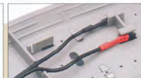
Wire attached to terminal
